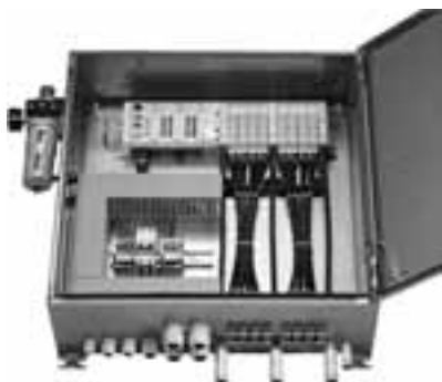
Customised control cabinet solution
